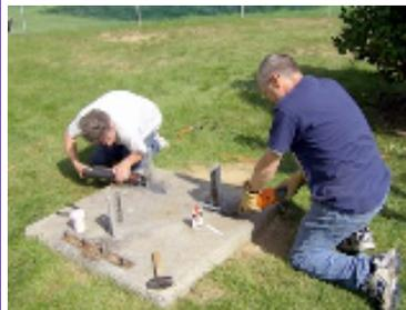
close to the concrete base with a combination of a die grinder and a reciprocating saw. Where the feedlines entered the house, we installed a new piece of vinyl over the
