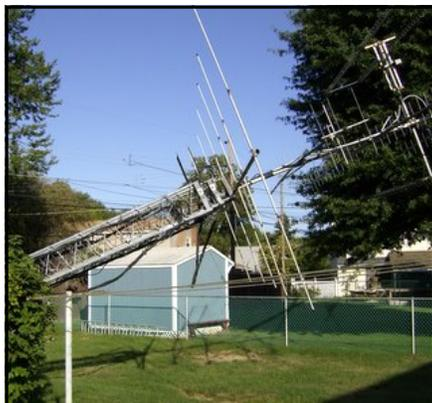
horizontal. Think of the tower as a giant lever. If the winch cable failed, the antennas might turn into so much scrap aluminum. **The cable held.**
